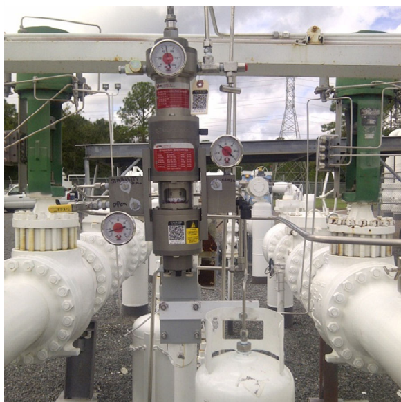
Figure 9 – VPC Replaces Bristol 624 VRG Controls shown above replaced Bristol 624-II Pressure Controller to provide improved pressure control performance in critical power plant fuel gas feed application. The VPC demonstrated more accurate control downstream pressure and eliminated sensitivity to vibration. VPC shown installed on Fisher 470 Series actuator with EWT Control Valve and 3610 Pneumatic Positioner.
