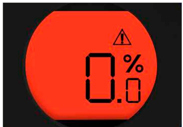
Fig 8.3 Actuator display flashes Red and White when RPP is active during power failure.
