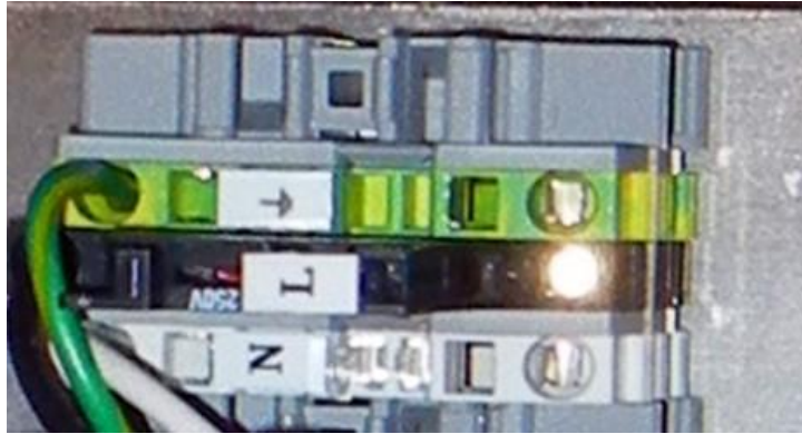
Figure (4.C.1)- power Terminal Blocks, AC Version
